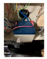
3. Remove each wire by gripping the wire close to the connector and gently pulling it off of the battery tab. If your alarm is not currently in a trouble condition, removing the battery will cause a trouble condition. This is normal. When the wires are removed, the battery will look like this:
